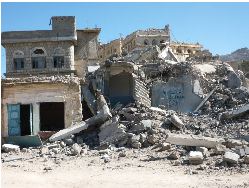
Building destroyed by aerial bombardment, Sa'dah, Yemen, March 2010 © Private
